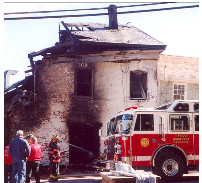
The William Valentine Store at 1 Tower Place was destroyed by fire in October 2001. (Photograph provided by John M. Collins.)
