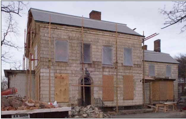
The HDB works to promote continued local preservation efforts in an effort to maintain its historic historical, cultural, architectural, archaeological, economic and social heritage for future generations of the Village of Roslyn's residents. In this case, removal of aluminum siding revealed historic wood shingles at the c.1804 Anderis Onderdonk House.
