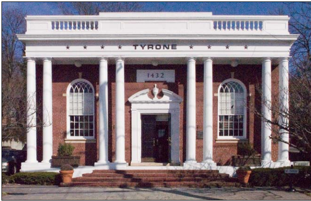
This former bank is now a clothing store.
